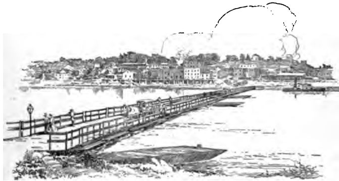
OLD PONTOON BRIDGE AT ST. CHARLES
